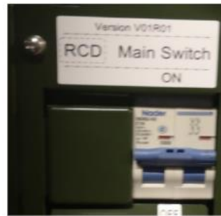
TNCS System with no RCD
