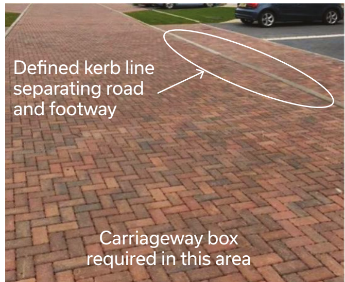
Example of a defined kerb line on a shared surface
