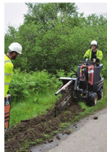
The ditch witch digger
